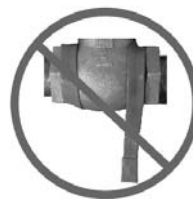
B.) Incorrect Installation: Heating tape hanging free from the surface
