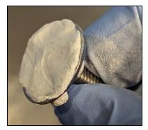
Figure 10: Completely cover bottom surface of stud with mixed epoxy
