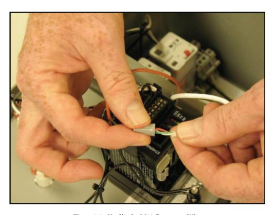
Figure 3-3. Unclip the M12 Connector Wire
