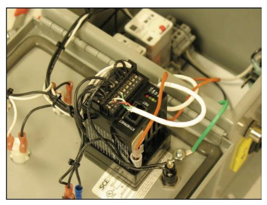
Figure 3-7. Place Wire Into Clip To Secure It. Close Box And Secure Box Cover Screws.
