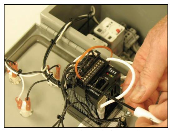
Figure 3-2. Remove The Thermocouple Wire From 1 and 2
